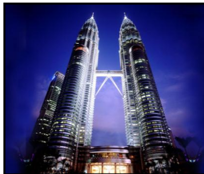
Petronas Twin Towers in KL
